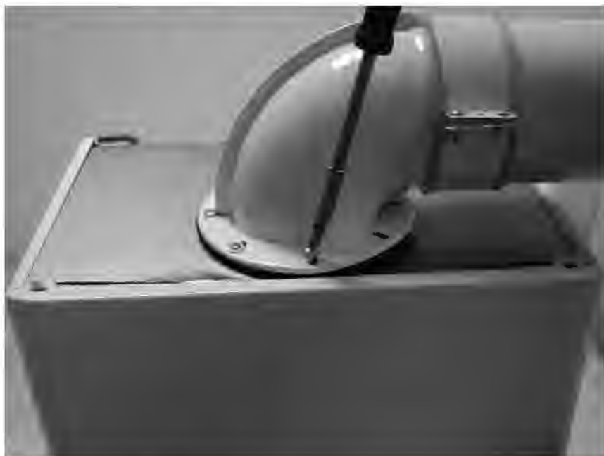
Picture13 : Remove the 4 star slotted screws attaching the flue to the appliance. After cracking the joint with a slight tap or twist the flue can be lifted clear of the appliance.
