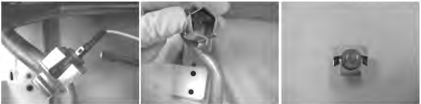
Picture 74 – 75 – 76 : Remove the electrical cable connections from the surface type NTC sensor, which is located on the surface of the hot water pipe, the NTC sensor used to fit onto the pipe surface can be easily removed from its bracket.
