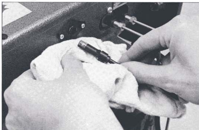
The photo cell is removed from burner for cleaning. Do not touch cell with the fingers and use only a clean dry cloth for cleaning. Ensure viewing face points towards burner combustion head when replacing.
